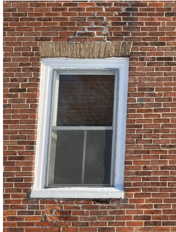
Plate 19: Main block window example
