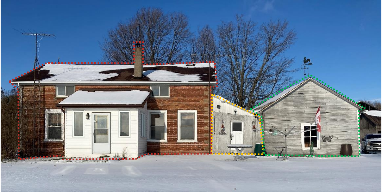
Plate 13: Front façade (east elevation) of the farmhouse, showing original main block (outlined in red), side passage (yellow), and summer kitchen (green).
