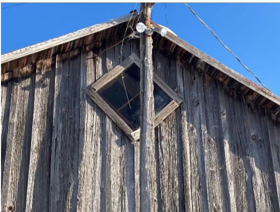
Plate 104: Diamond gable window on south elevation of Outbuilding No. 1
