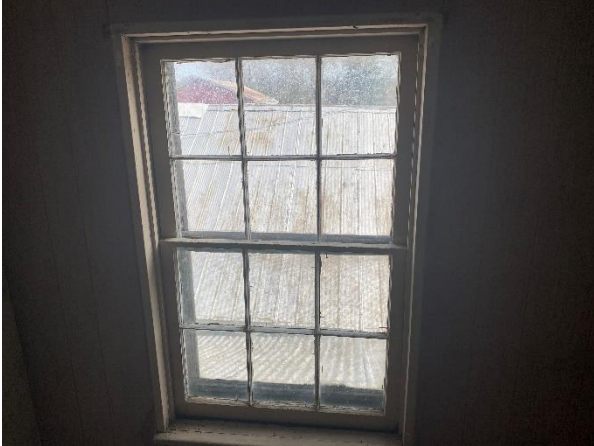
Plate 52: Six-over-six sash window in northeast bedroom
