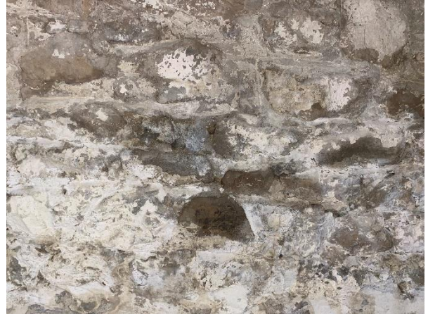
Plate 34: Parged stone foundation
