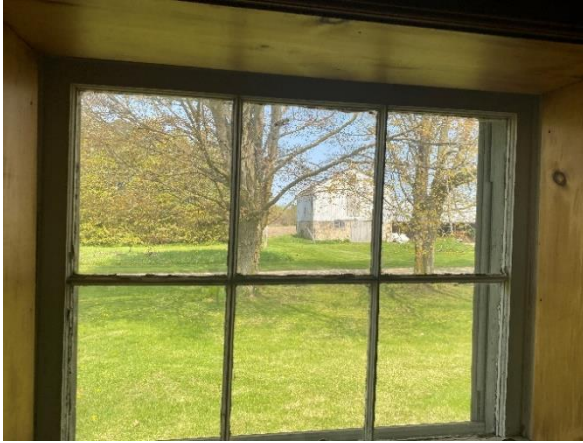
Plate 71: West elevation window
