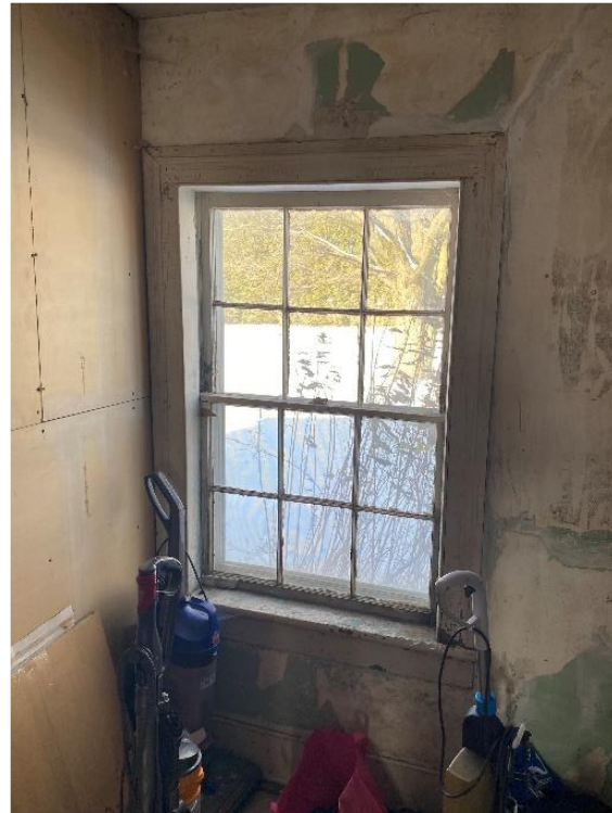
Plate 74: Rear addition storage room window on west elevation
