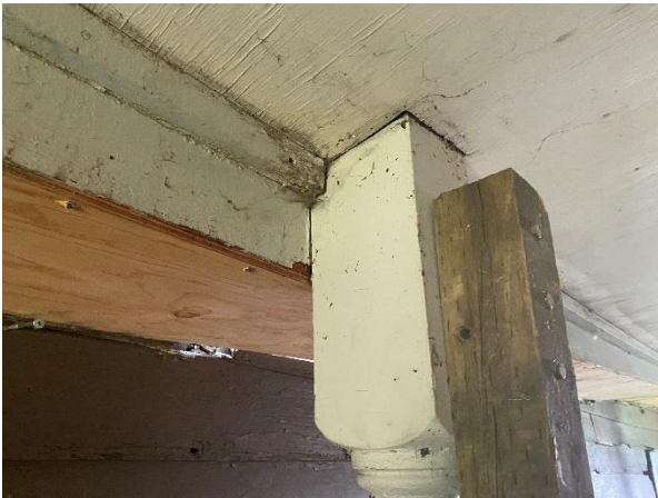
Plate 79: Original veranda pillar
