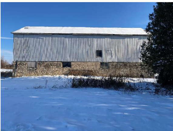
Plate 92: South elevation of south barn
