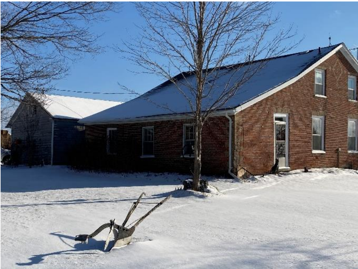
Plate 64: Oblique view of side addition
