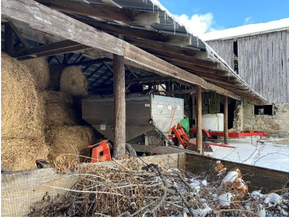
Plate 100: Junction between connecting shed and north barn
