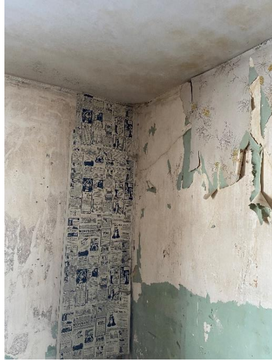
Plate 72: Rear addition storage room
