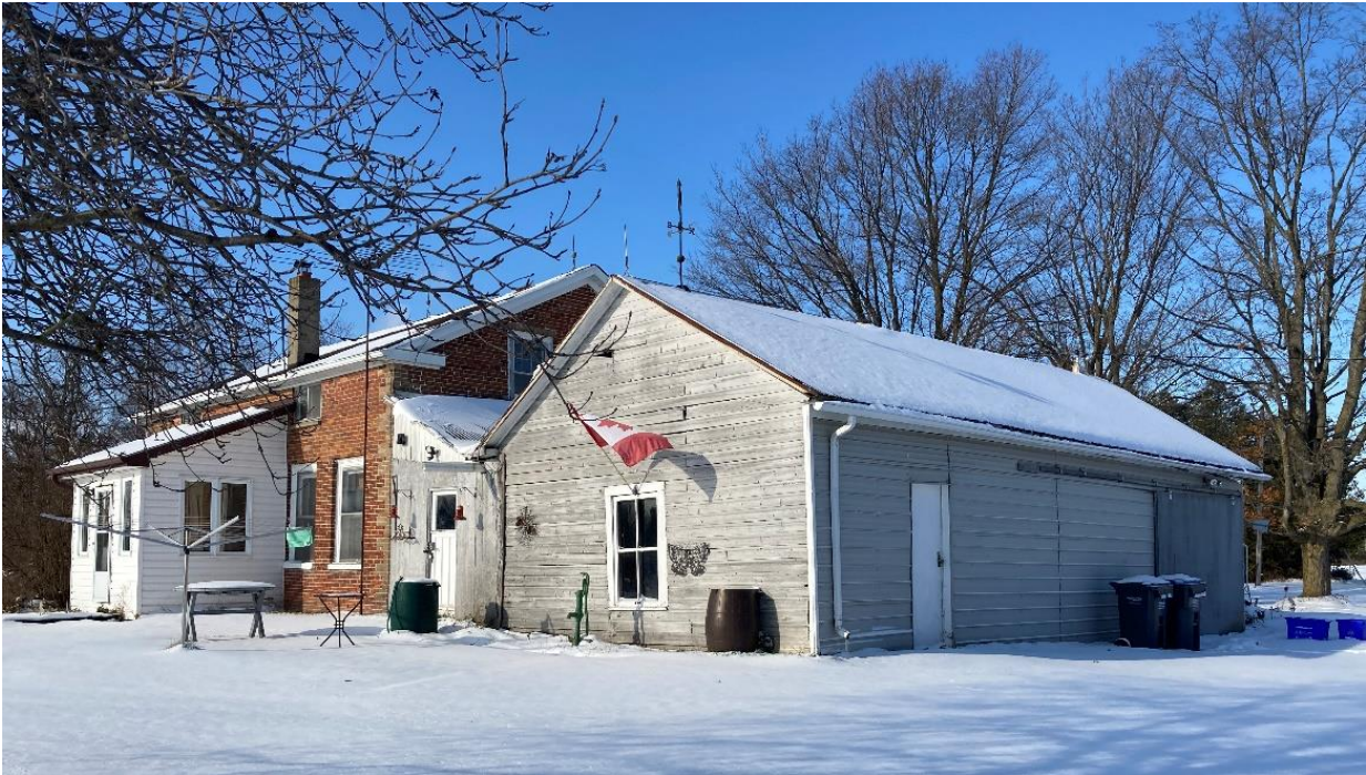
Plate 16: Oblique view of east (left) and north (right) elevations
