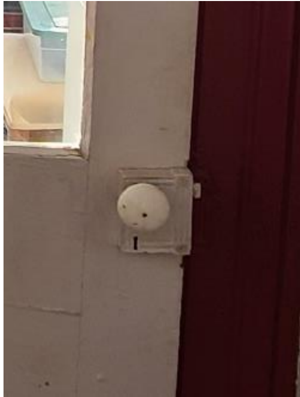
Plate 27: Rim lock detail of east entry door
