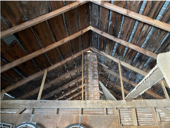
Plate 85: Central brick chimney remnant in summer kitchen
