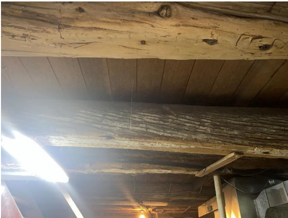
Plate 35: Hand hewn log floor joists
