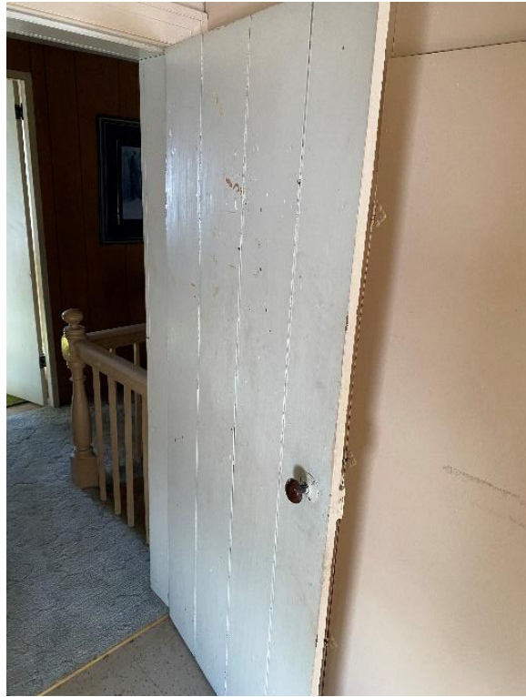
Plate 57: Vertical panel door to northeast room
