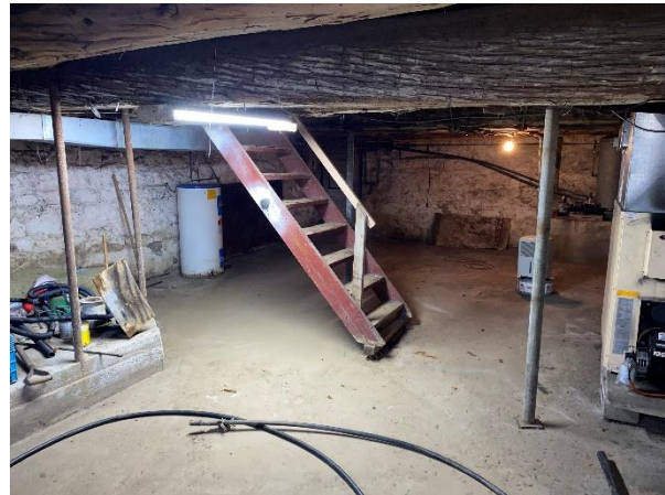
Plate 32: Basement of the farmhouse
