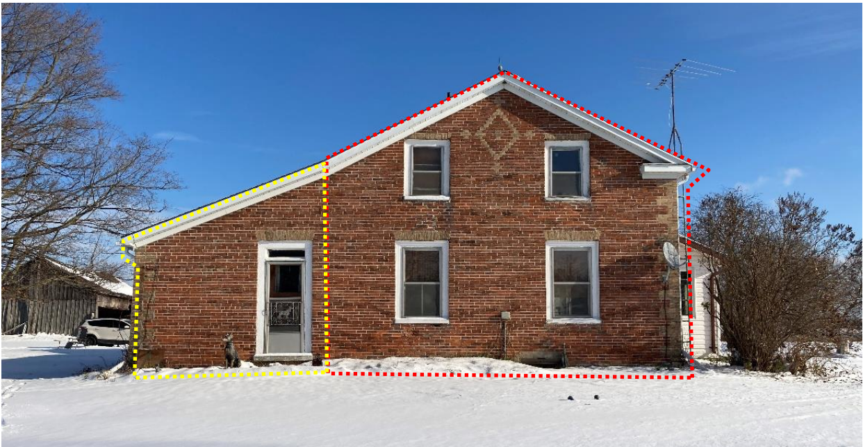
Plate 14: South elevation, original main block is outlined in red, rear addition is outlined in yellow
