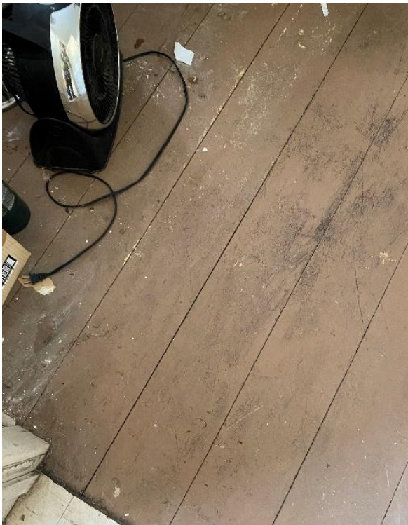
Plate 73: Wood floors of Rear addition storage room
