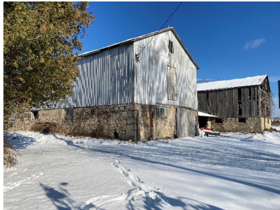
Plate 89: South and east elevations of the H-shaped barn complex
