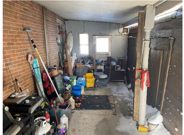
Plate 78: Enclosed frame and plywood side passage on the north elevation
