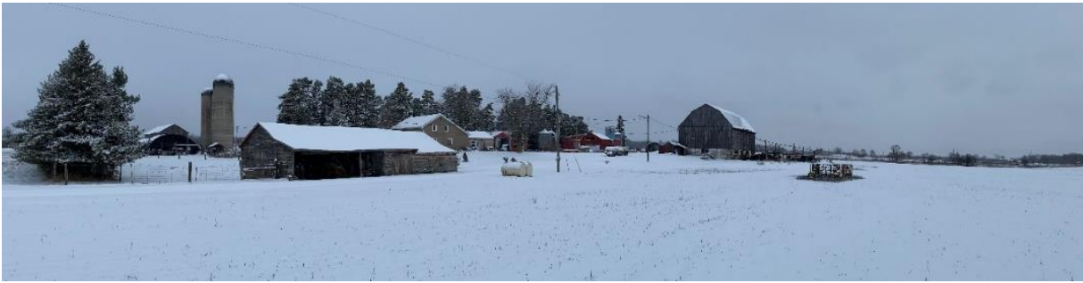
Plate 4: Farm complex at 18501 Mississauga Road (Listed on the Town of Caledon's heritage register)
