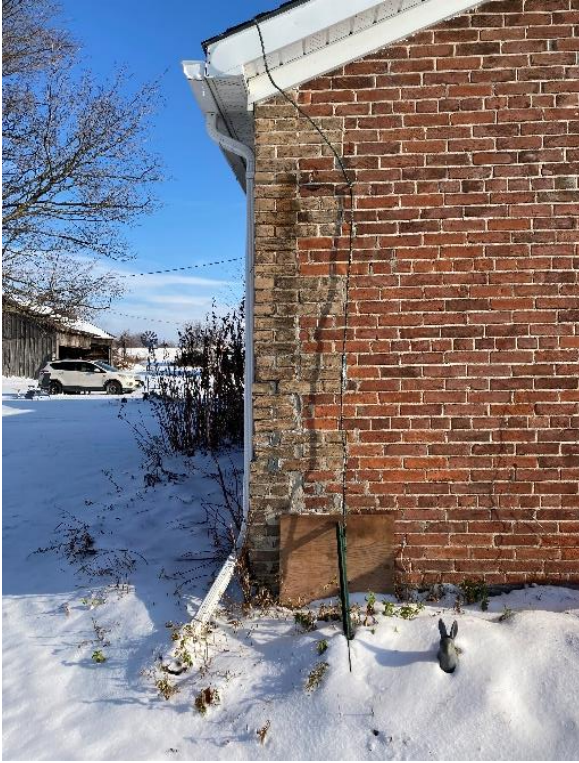
Plate 65: Detail of southwest corner, showing quoins
