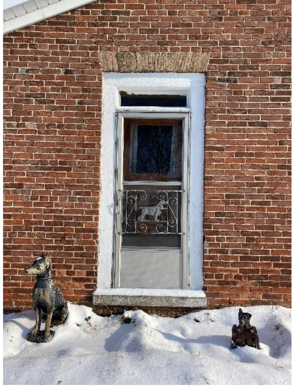
Plate 66: South elevation entrance
