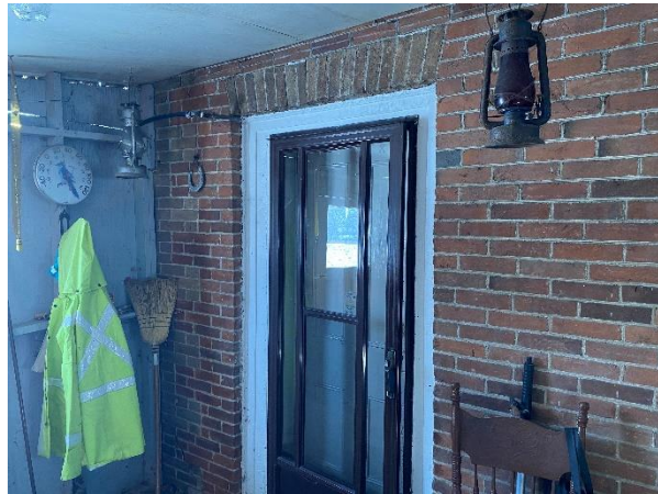
Plate 29: North elevation entrance
