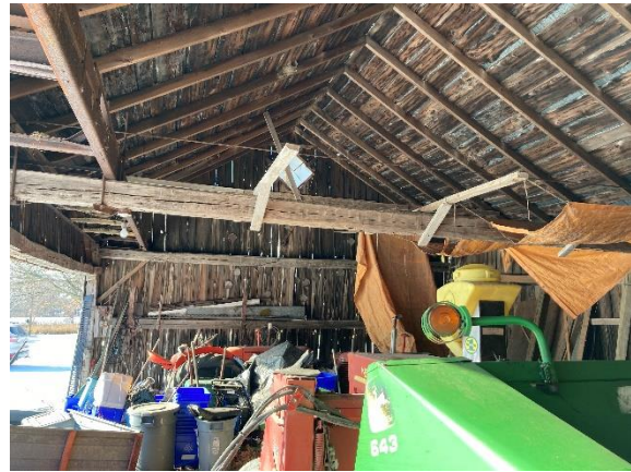
Plate 103: Interior of Outbuilding No. 1
