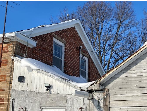
Plate 28: Portion of north elevation of original main block visible from exterior
