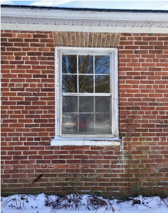
Plate 67: West elevation window
