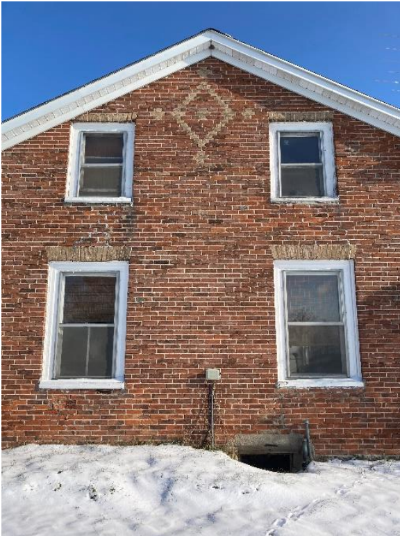
Plate 18: South elevation of main block
