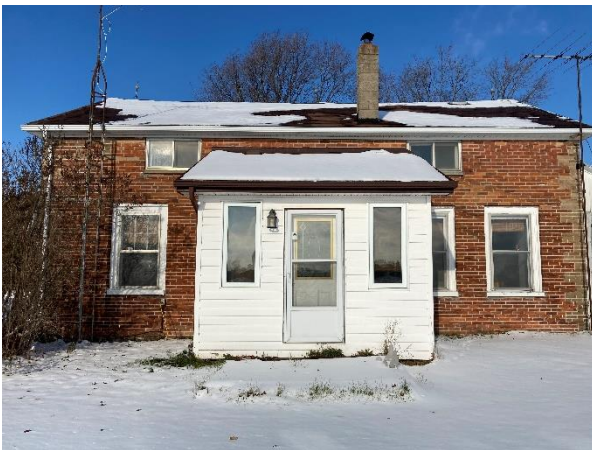
Plate 24: Porch entry on east elevation (original front façade)
