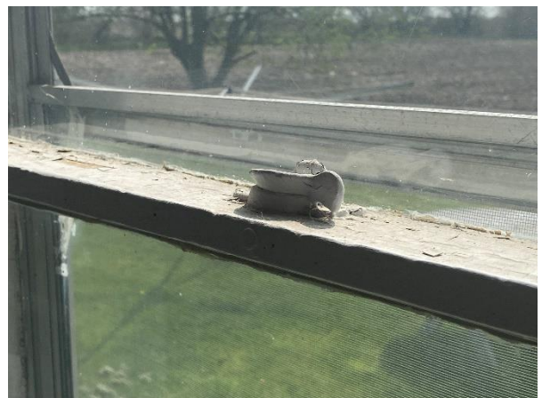
Plate 44: East elevation window
