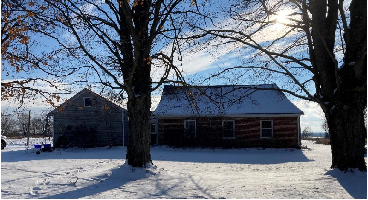
Plate 17: West elevation of the farmhouse
