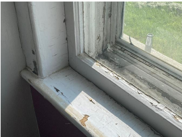
Plate 43: East elevation window
