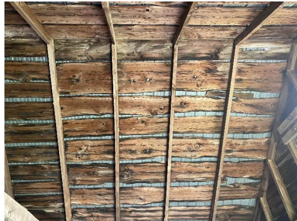
Plate 87: Wide board roof sheathing
