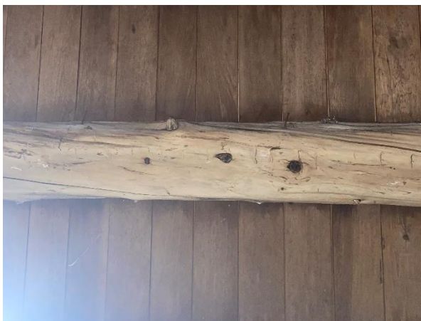
Plate 37: Main block plank subflooring
