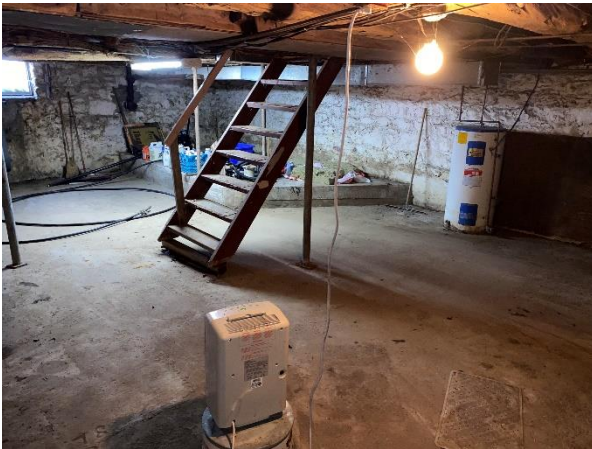
Plate 31: Basement of the farmhouse
