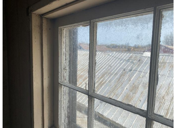
Plate 53: Detail of six-over-six sash window in northeast bedroom
