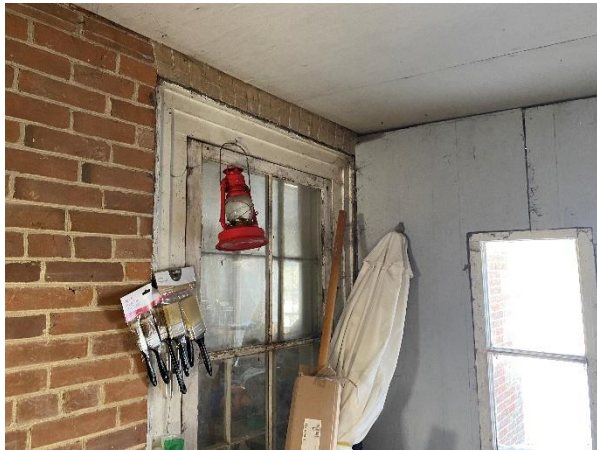
Plate 68: North elevation window
