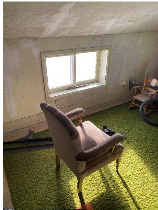
Plate 51: East window of southeast second floor room
