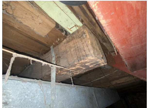
Plate 36: Hand squared floor joist
