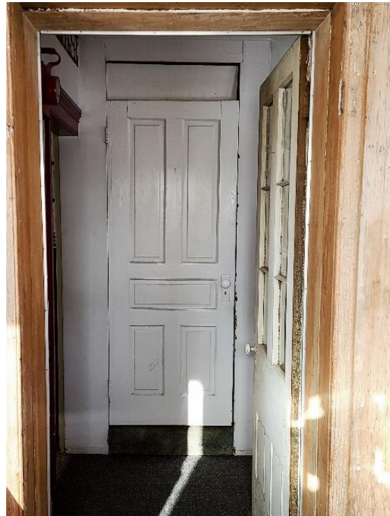
Plate 47: Five panel door leading to the second floor
