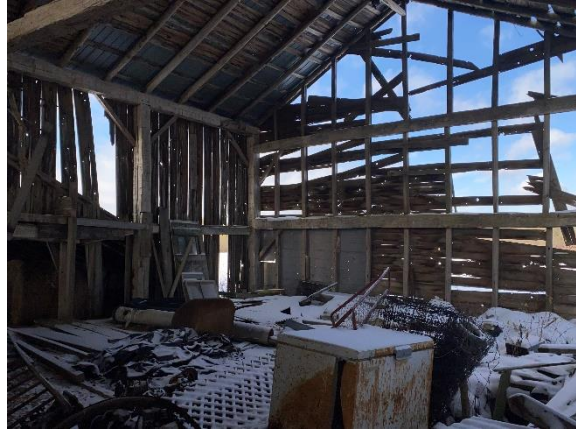
Plate 95: North barn interior showing hand hewn beams
