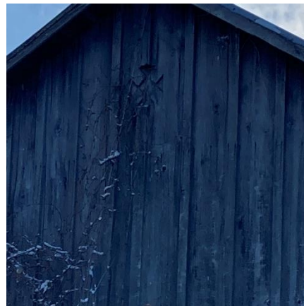
Plate 105: Diamond cross owl hole on north elevation of Outbuilding No. 1
