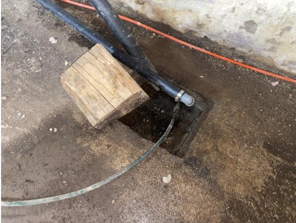
Plate 33: Poured concrete basement flooring
