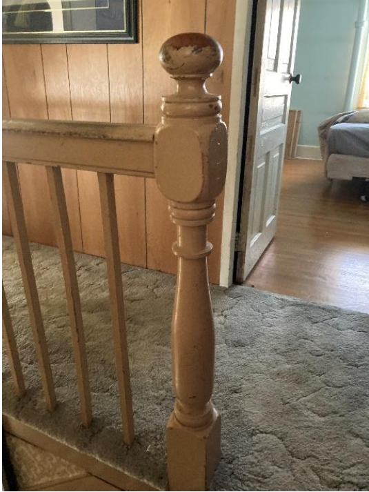
Plate 48: Newel post, handrail, and balustrade of second floor
