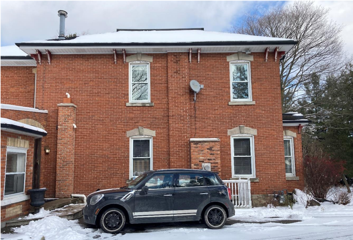
Plate 20: South portion of the west elevation of original main block
