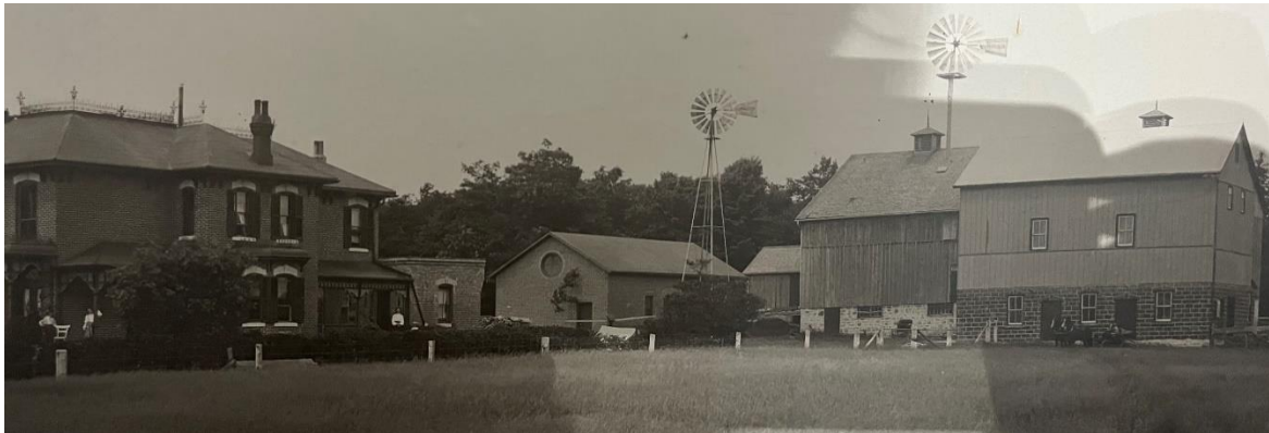
Plate 1: Historical photograph of the house and outbuildings, date unknown.
