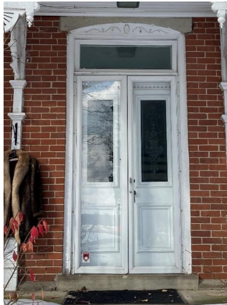
Plate 27: Main entrance doorway (south elevation)
