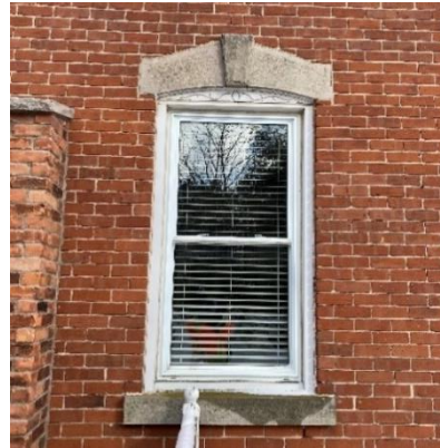
Plate 23: Main block window example
