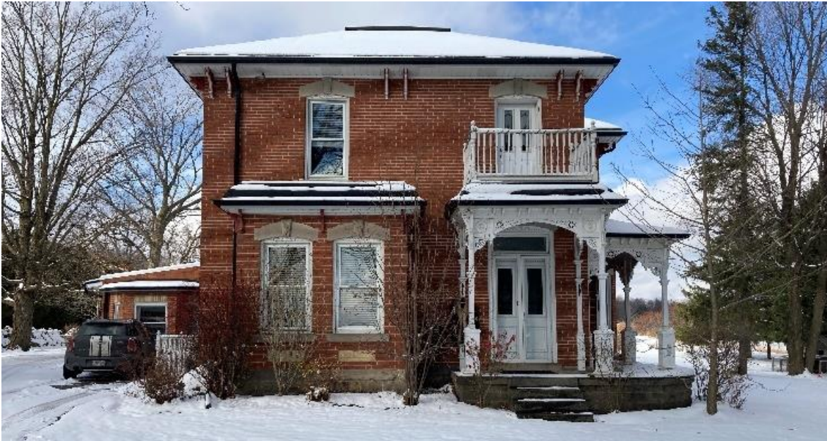
Plate 16: South (front) elevation, facing Charleston Sideroad
