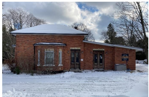
Plate 42: North elevation of rear/side addition
