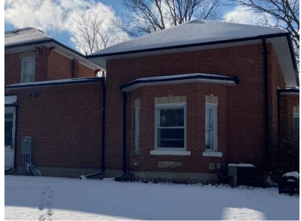
Plate 44: Detail of east elevation bay window
