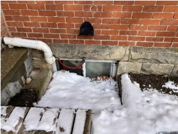
Plate 24: Cut stone foundation
