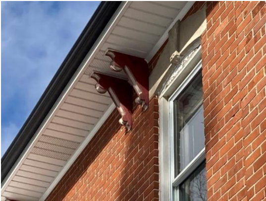
Plate 22: Overhanging eaves and paired bracket detail
