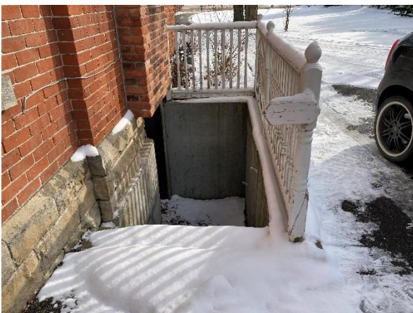
Plate 38: Basement access on west elevation
