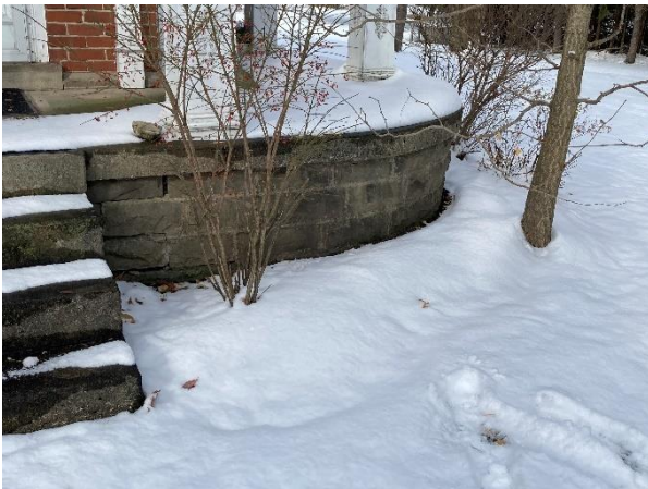
Plate 30: Stone foundation of the front and side porches
