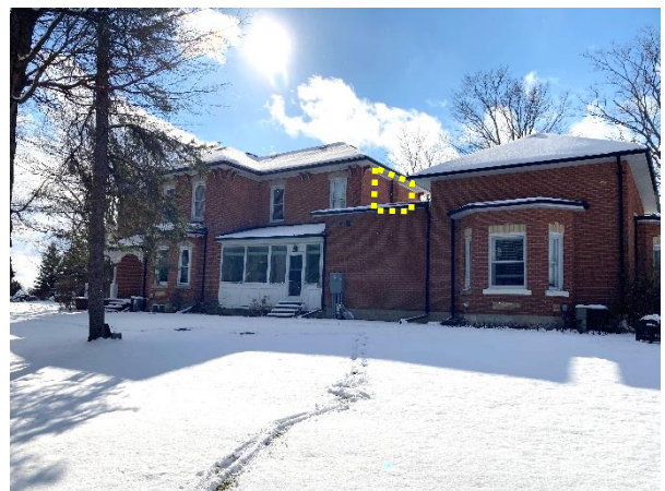
Plate 39: East elevation with former external chimney visible on original main block (highlighted in yellow)
