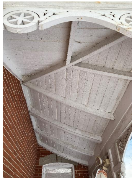
Plate 31: Bellcast roof of the side porch
