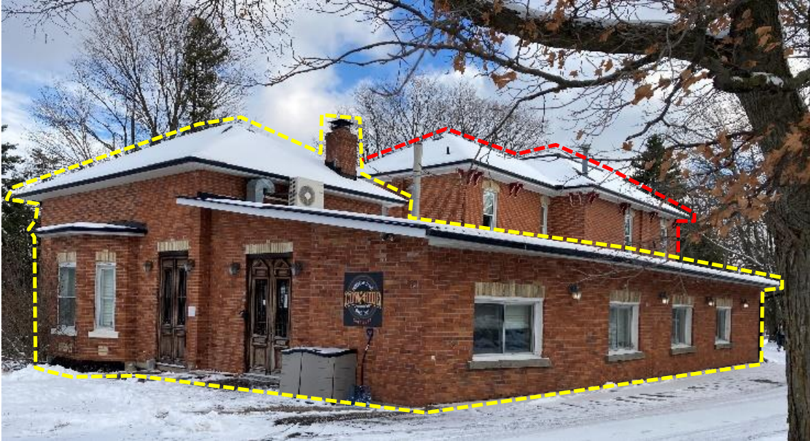
Plate 19: Oblique view of north and west elevations of rear and side additions (outlined in yellow, original main block is outlined in red)
