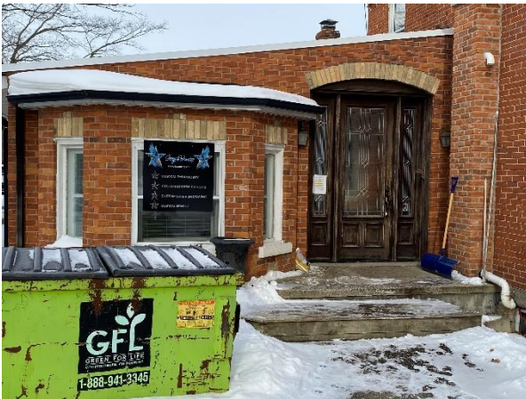
Plate 45: South entrance to side addition
