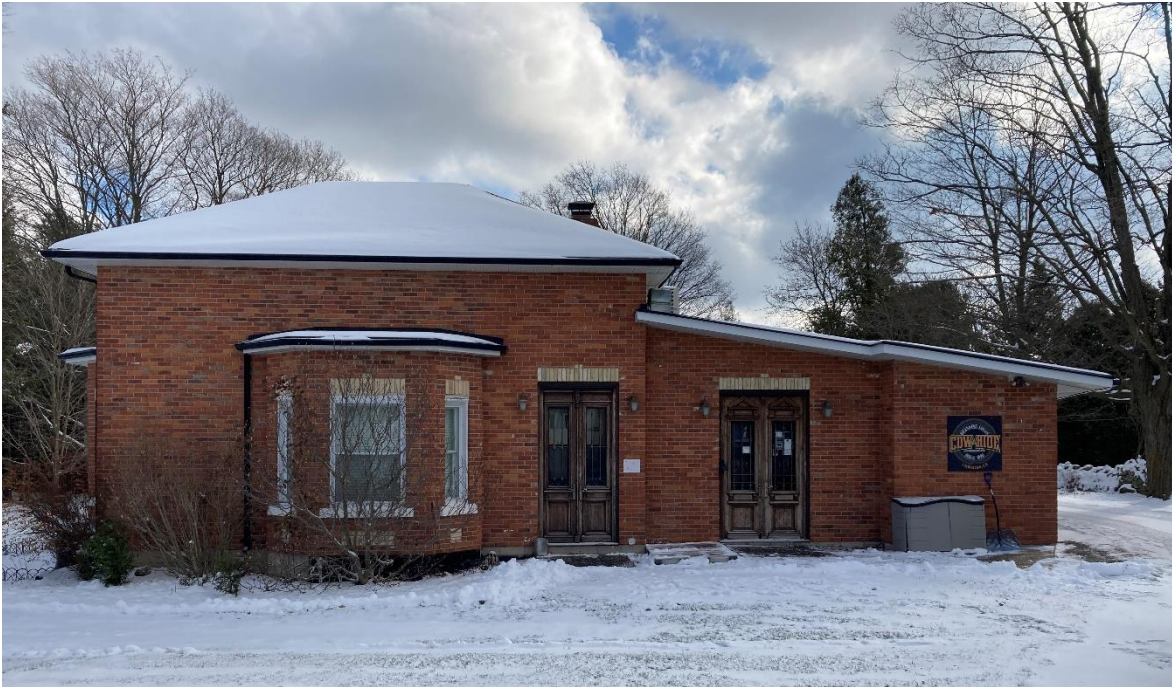
Plate 18: North (rear) elevation (rear and side addition visible only)
