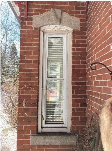
Plate 26: Detail of box bay side windows
