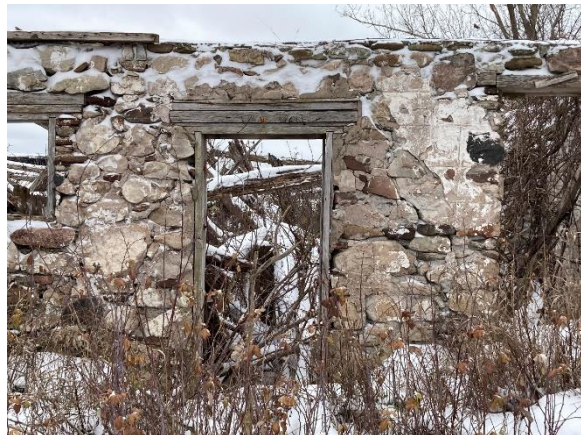
Plate 22: Parged fieldstone wall and doorway
