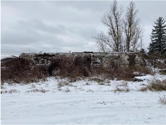
Plate 19: West elevation of Structural Foundation No. 1
