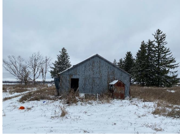
Plate 16: South elevation of outbuilding
