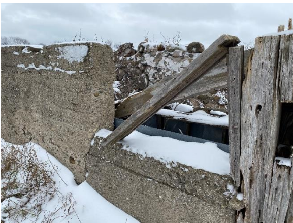
Plate 30: Wood fenestration elements of Structural Foundation No. 2
