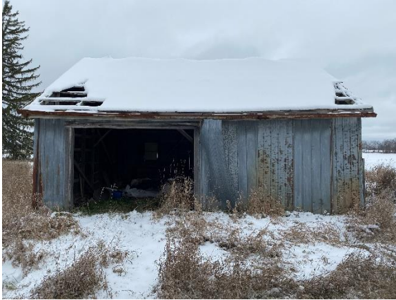
Plate 15: West (front) elevation of outbuilding
