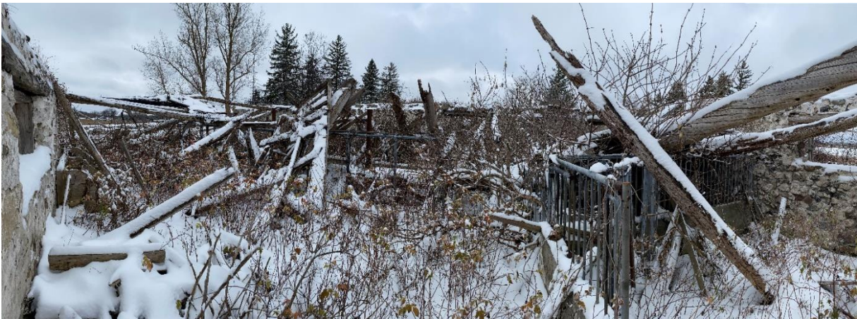
Plate 27: Panoramic photo of Structural Foundation No. 1 interior
