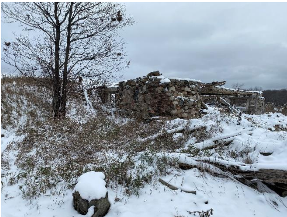
Plate 21: Earthen ramp north of Structural Foundation No. 1
