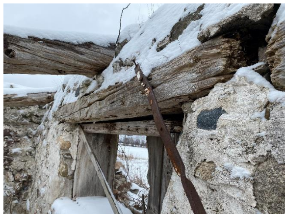
Plate 24: Wood lintel and frame
