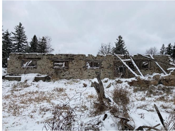
Plate 20: South elevation of Structural Foundation No. 1
