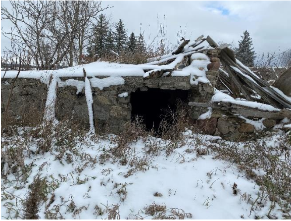
Plate 32: Entrance to below grade cellar
