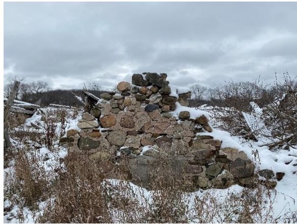
Plate 29: Parged fieldstone walls of Structural Foundation No. 2
