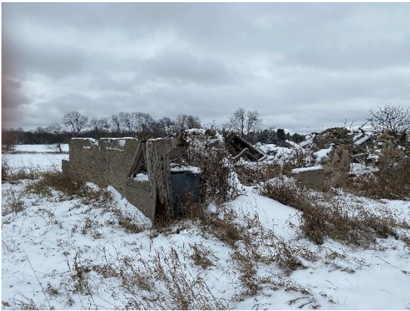
Plate 28: Concrete walls of Structural Foundation No. 2
