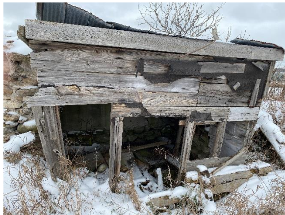
Plate 31: Wood lean-to addition
