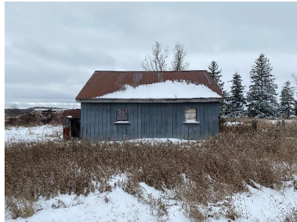
Plate 18: East elevation of outbuilding
