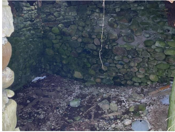
Plate 33: Fieldstone wall of below grade cellar interior
