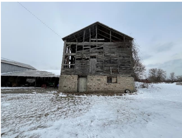
Plate 45: East elevation of the North Barn
