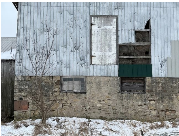
Plate 26: Windows in the fieldstone foundation
