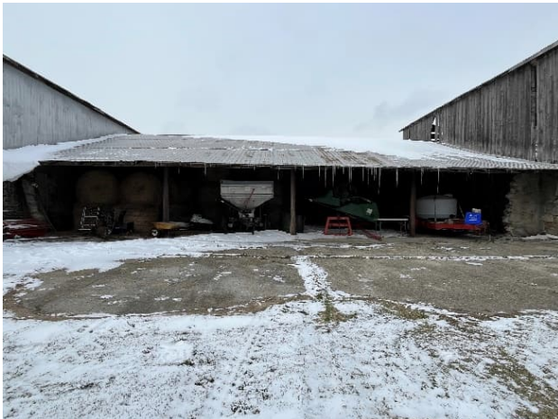
Plate 36: East elevation of the Connecting Shed
