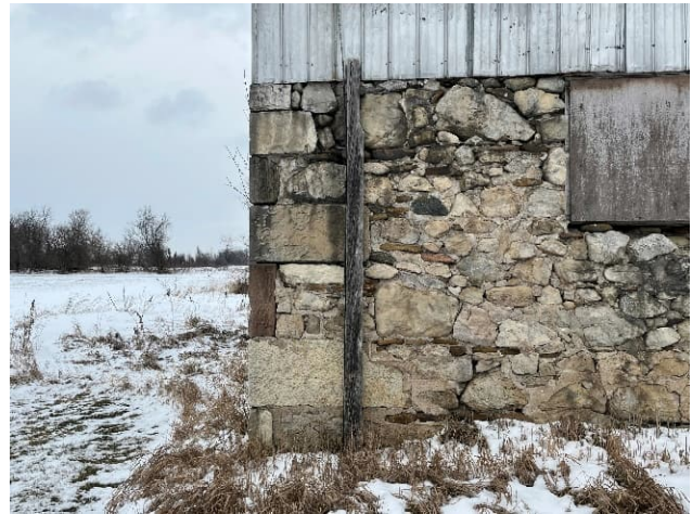
Plate 21: Cut stone quoining
