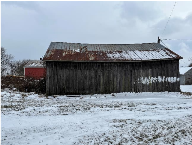
Plate 61: West elevation of the Drive Shed
