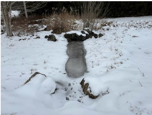
Plate 13: Creek running under the driveway
