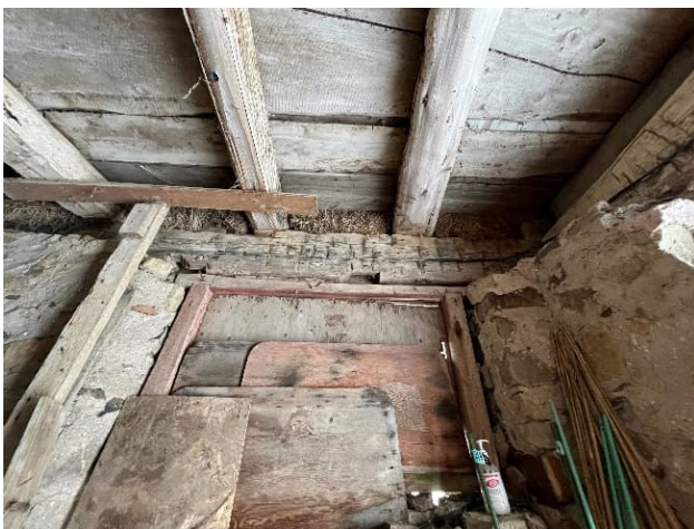
Plate 32: Hand-squared sill with redundant mortises supporting log joists
