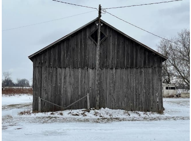
Plate 60: South elevation of the Drive Shed
