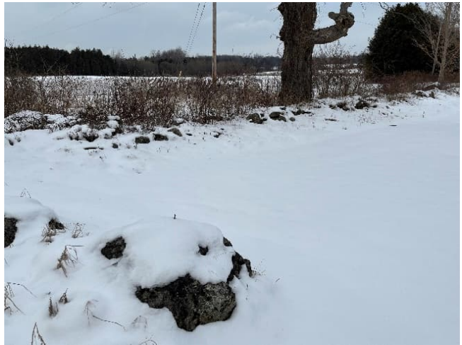
Plate 68: Portion of the fieldstone wall on the west side of the driveway
