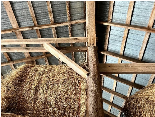
Plate 38: Recycled timber posts paired with dimensional lumber framing
