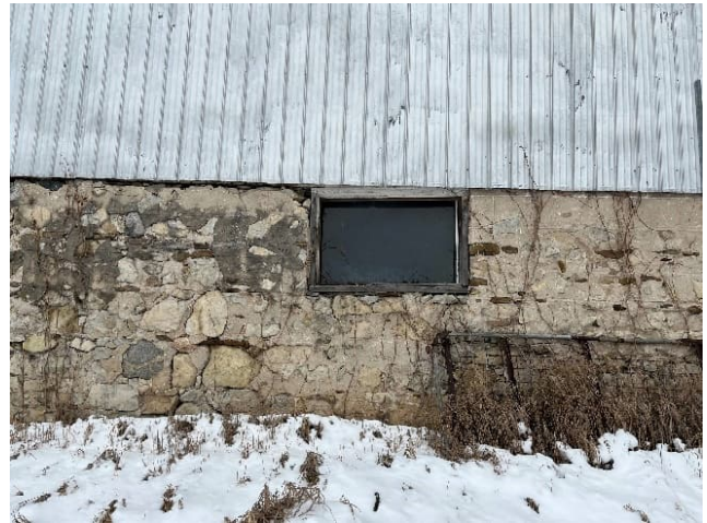
Plate 23: Window on the south elevation
