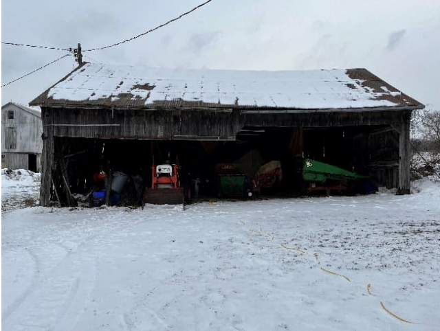
Plate 59: East elevation of the Drive Shed
