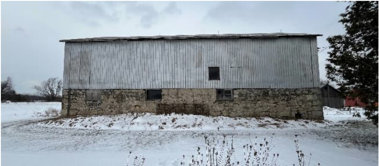
Plate 19: South elevation of the South Barn
