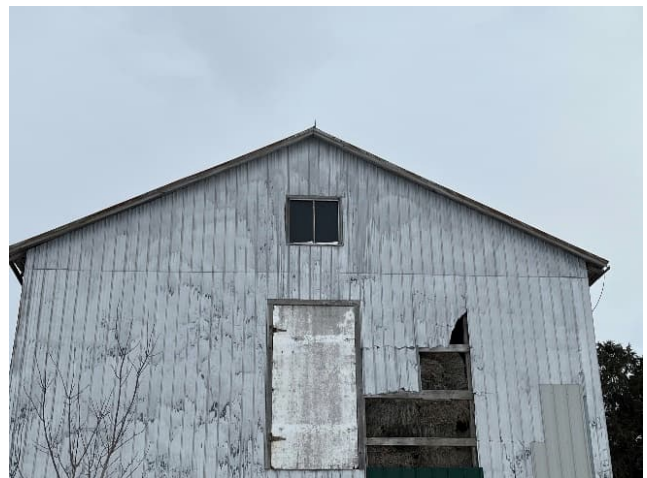
Plate 27: Upper-level door, exposed framing, gable window
