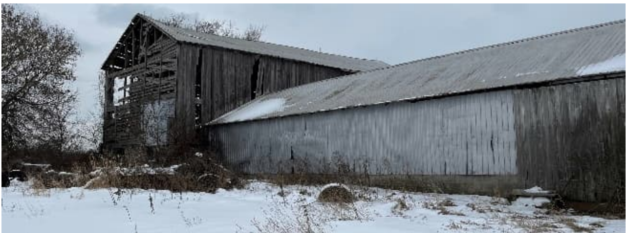
Plate 42: West elevation of the Connecting Shed
