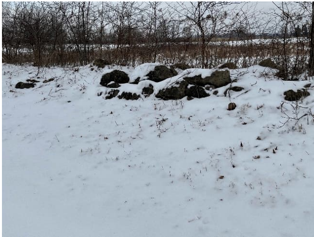
Plate 67: Portion of the fieldstone wall on the east side of the driveway
