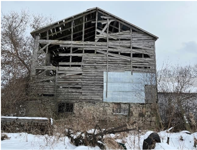
Plate 53: West elevation of the North Barn
