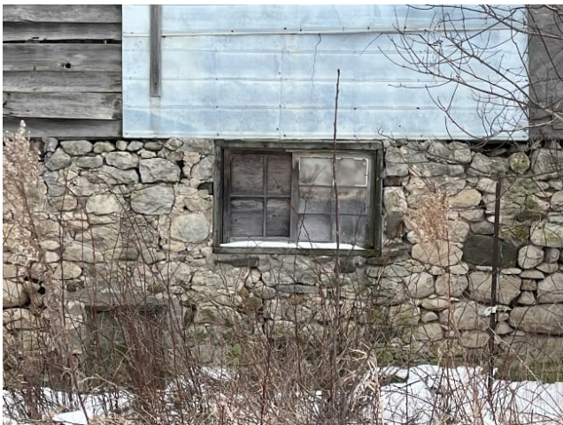
Plate 55: Paired windows on the south side of the west elevation
