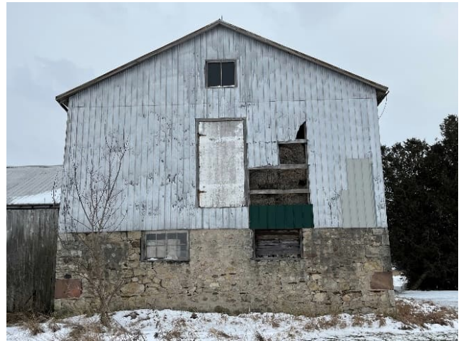
Plate 25: West elevation of the South Barn
