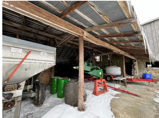
Plate 37: Open bays of the Connecting Shed
