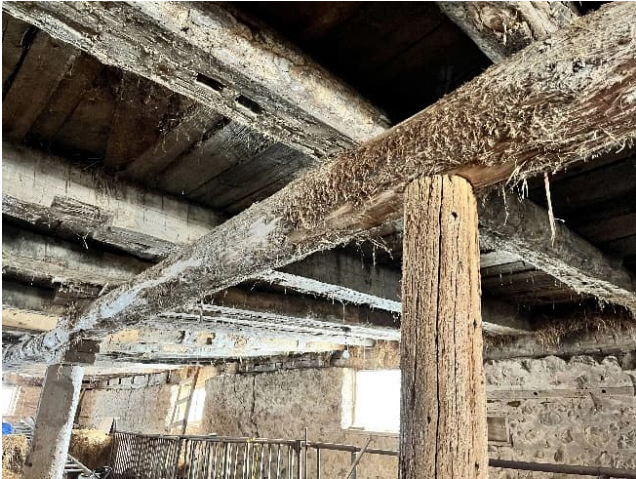
Plate 34: Redundant mortices in the hand squared joists
