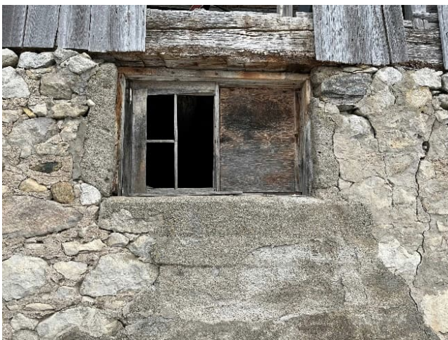
Plate 57: Partially blind paired window
