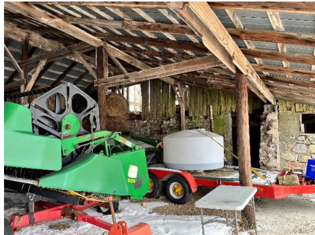
Plate 39: Wood posts and dimensional lumber framing
