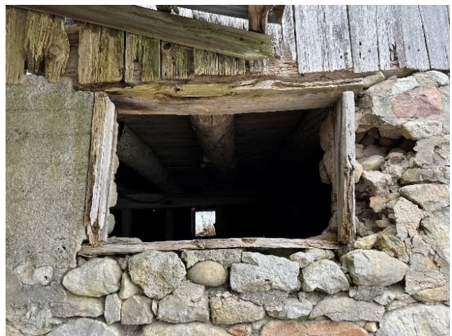
Plate 58: Wood framed window opening
