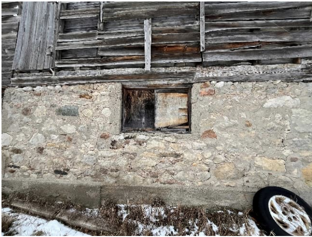
Plate 47: Blind window on the east elevation
