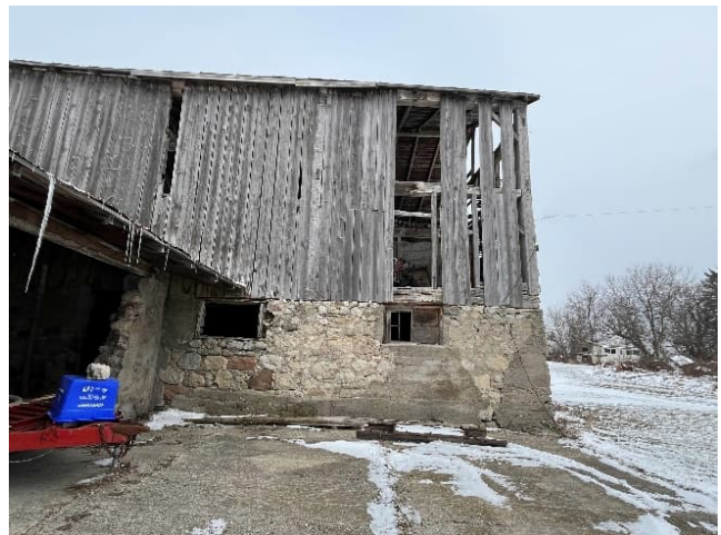
Plate 56: South elevation of the North Barn
