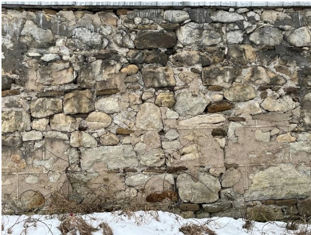
Plate 20: Partially parged fieldstone foundations
