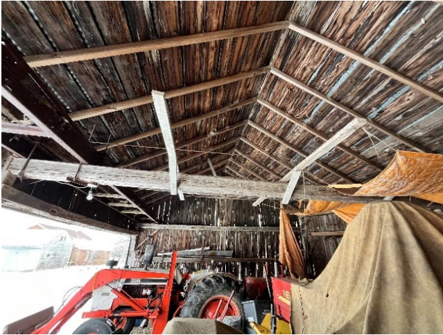
Plate 63: Wide plank sheathing on rafters
