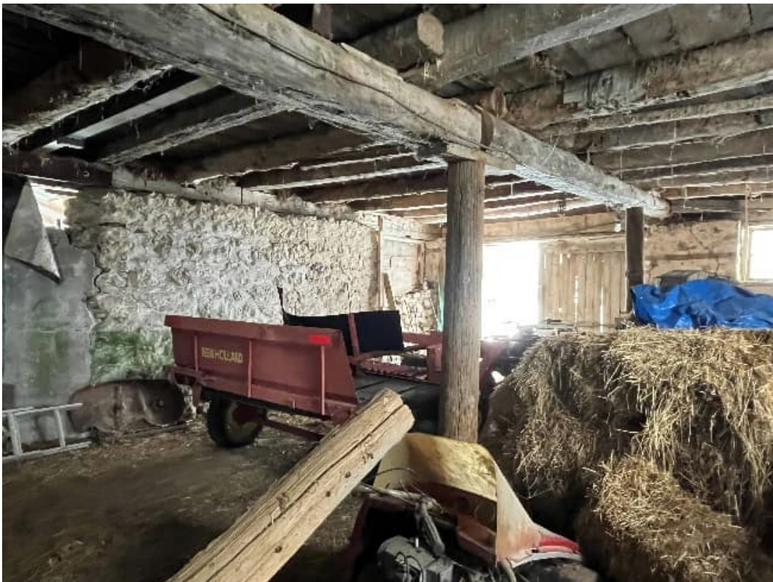
Plate 30: Lower level interior
