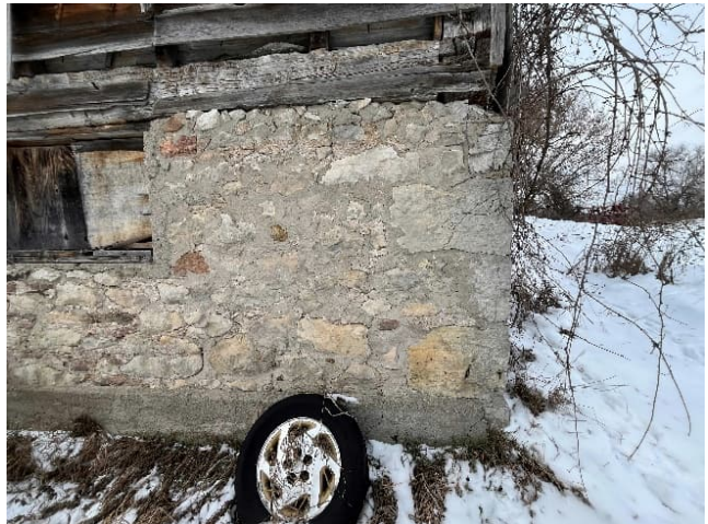
Plate 48: Irregular cornerstones on the east elevation
