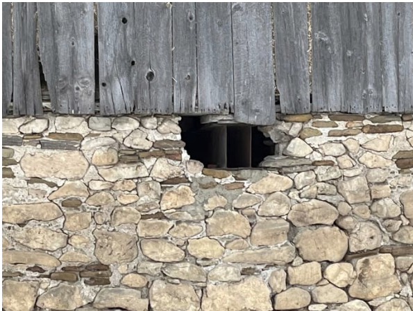
Plate 23: Hole in the foundation where a metal I-beam has been installed
