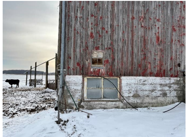
Plate 47: Window on the east side of the north elevation
