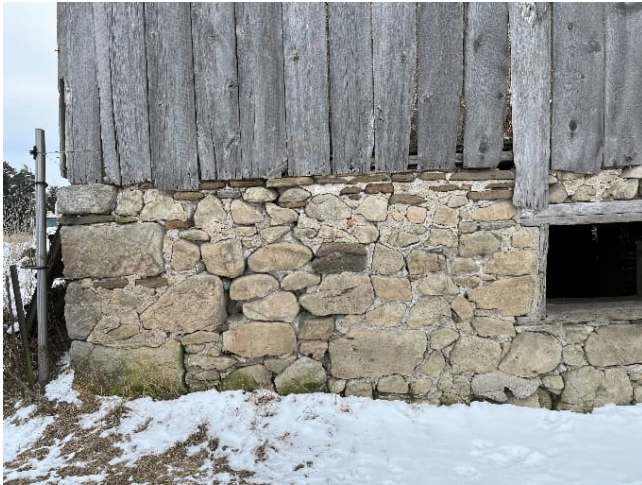
Plate 21: Fieldstone foundation on the northwest elevation
