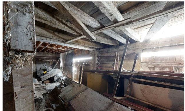
Plate 32: Storage room located at the south side of the barn
