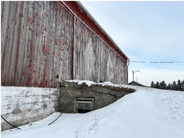
Plate 46: Gangway leading to the main entrance with window in the wing wall
