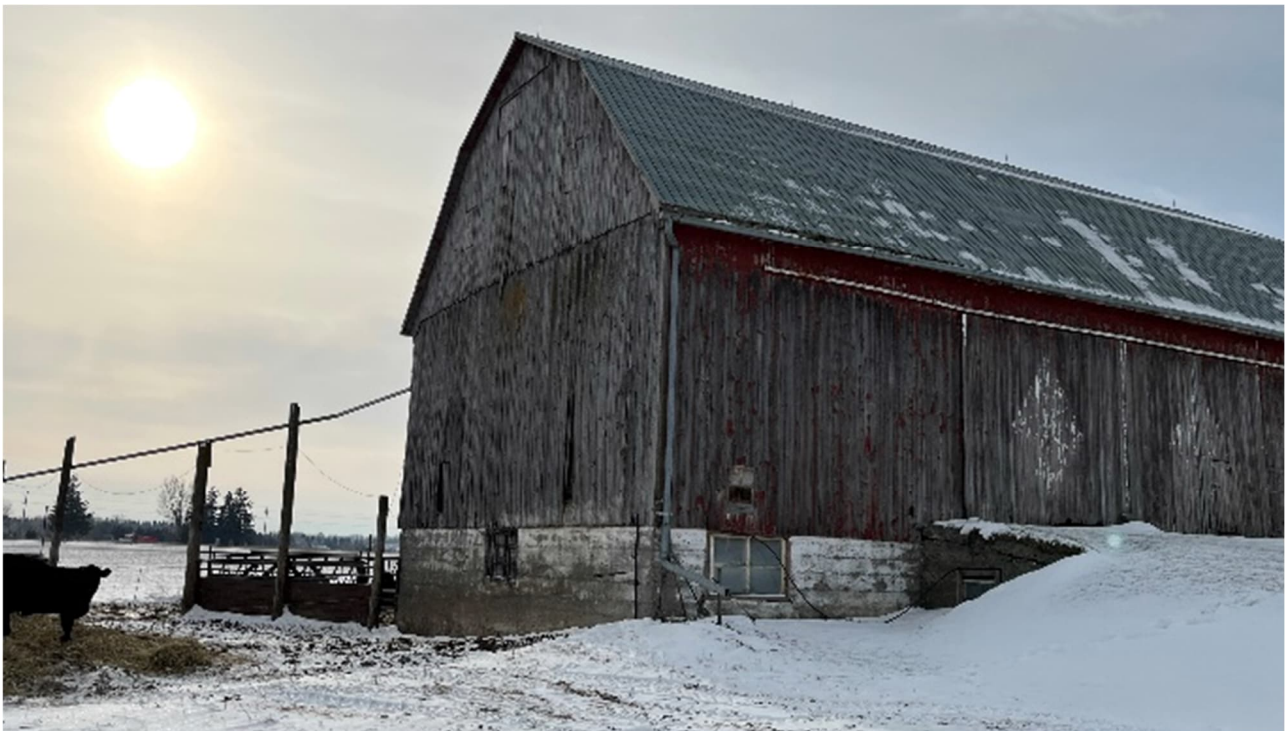
Plate 40: East elevation of Barn No. 2
