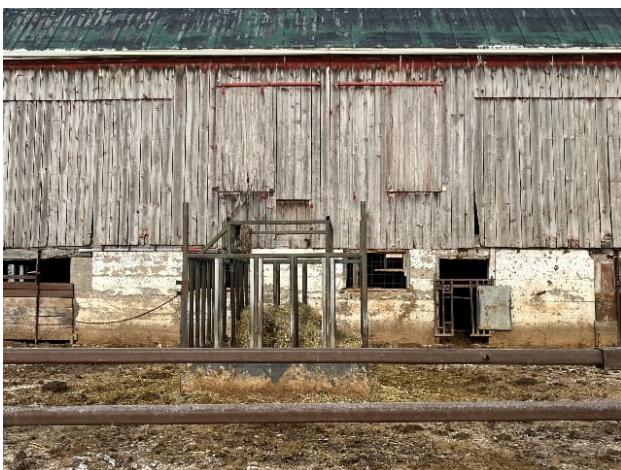
Plate 48: Windows and barred entrance on the south elevation
