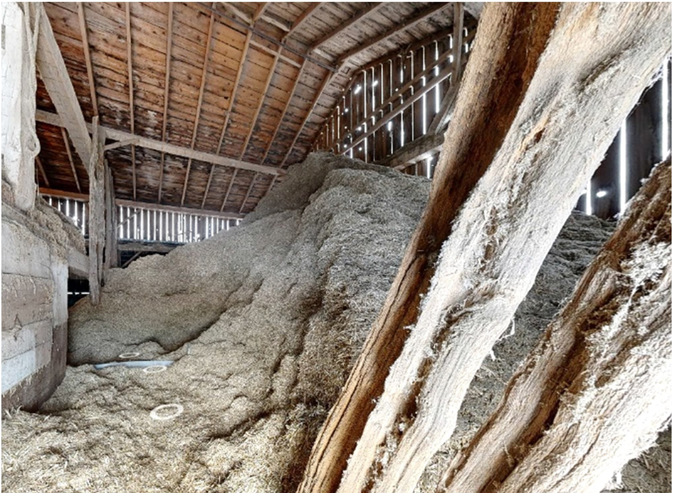
Plate 29: View of the rear side of the barn interior
