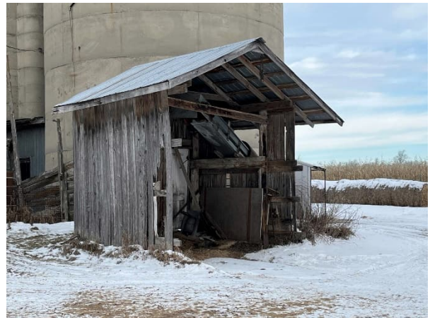
Plate 28: Gable roofed shed near silos
