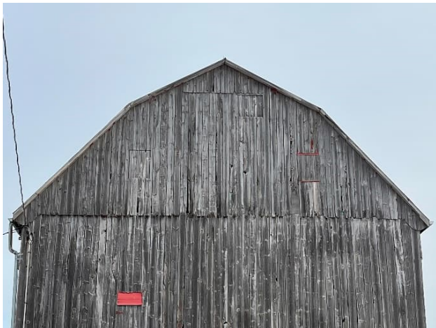
Plate 42: Gambrel roof of Barn No. 2
