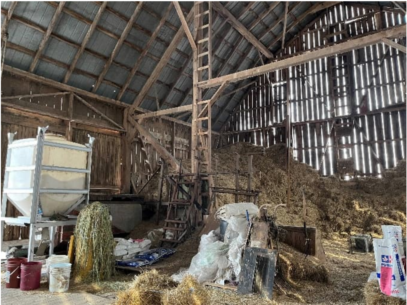
Plate 52: Upper level of Barn No. 2, looking northeast
