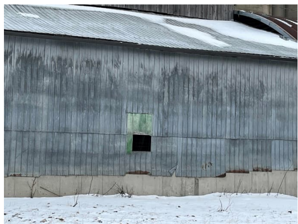
Plate 26: Southwest addition fiberglass windows
