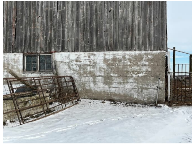
Plate 43: Cast-in-place concrete foundation and vertical wood plank siding
