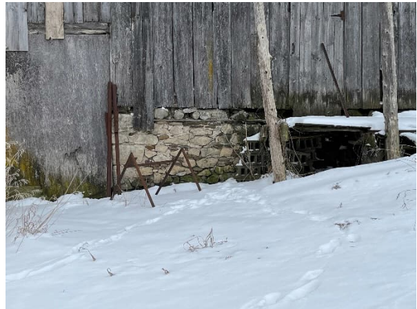
Plate 24: Fieldstone foundation seen on the northeast elevation
