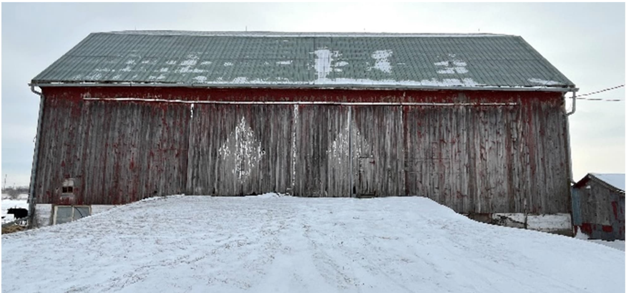
Plate 39: North elevation of Barn No. 2
