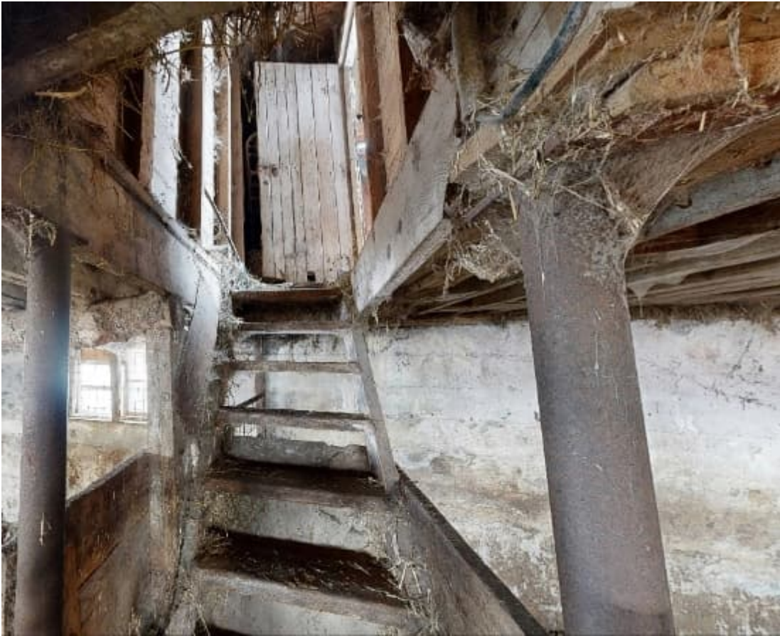
Plate 55: Stairs between upper and lower levels of Barn No. 2
