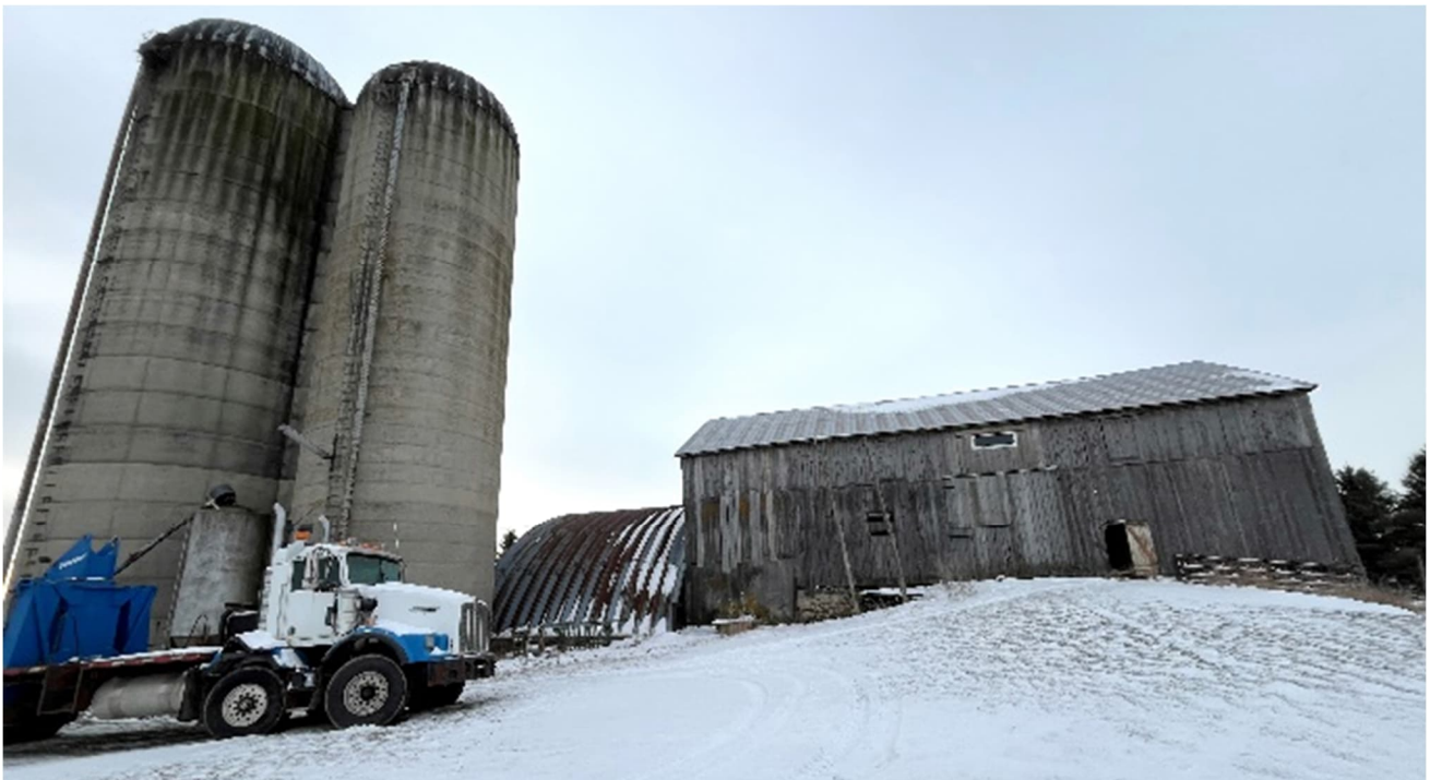
Plate 16: East elevation of Barn No. 1 (barn outlined in red, Quonset outlined in yellow)
