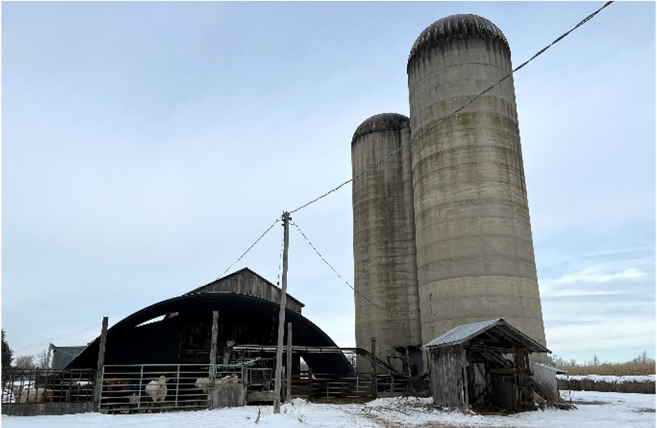
Plate 15: South elevation of Barn No. 1 (barn outlined in red, Quonset addition outlined in yellow)
