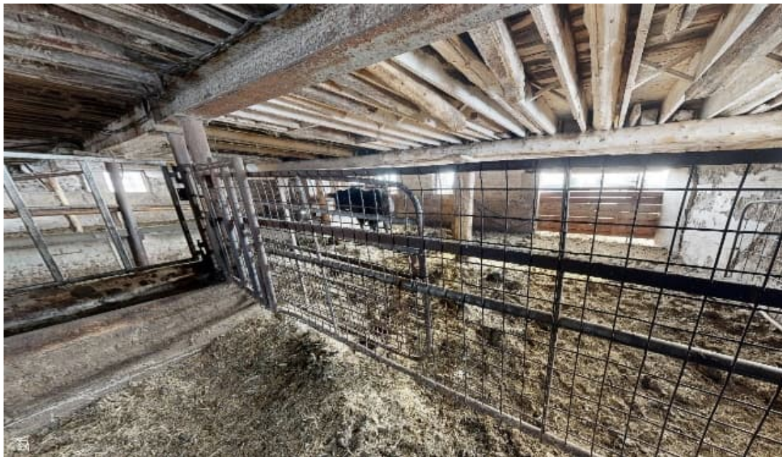
Plate 56: Lower level of Barn No. 2
