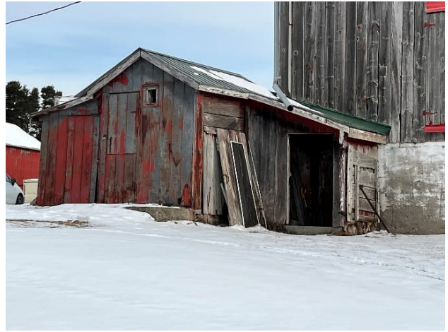
Plate 45: Metal clad shed at the northwest corner of Barn No. 2
