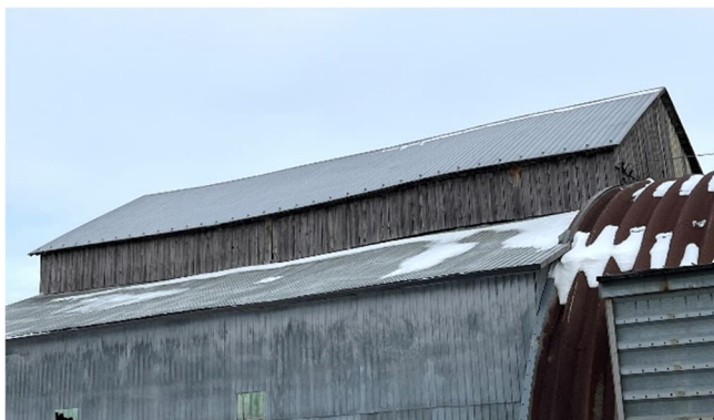
Plate 19: Gable roof seen behind the west addition
